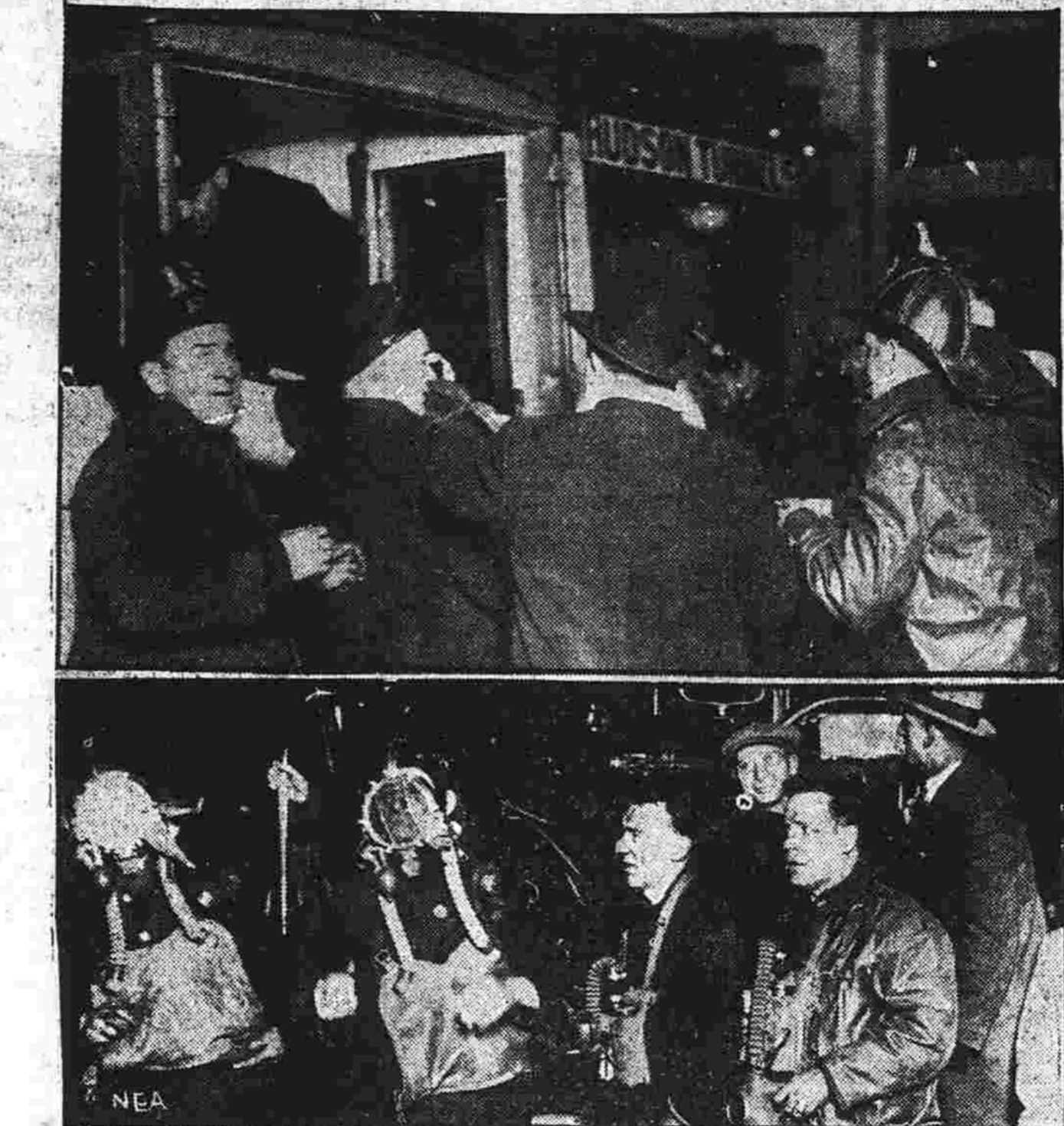
A seven-car train, jammed with commuters home ward bound for Jersey City, N. J., sped through a tube under the Hudson River. Suddenly the tunnel was filled with sickening smoke. The train stopped. Lights went out. Flames cracked. One of the seven cars had caught on fire. Fifty were injured and hundreds overcome in a scene of panic in the darkness underground. Above you see one of the victims being placed in an ambulance at an entrance to the tube. Below are firemen, gas-masked and begrimed, as they emerged from the smoke-filled tunnel after their rescue work.
